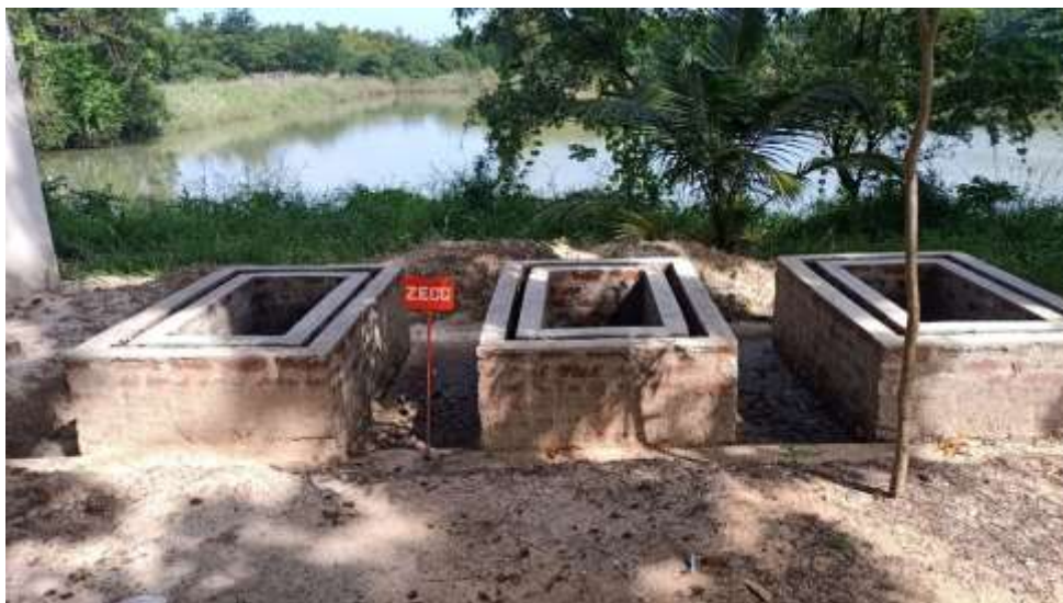
Grading and Washing Facility and ZECC
