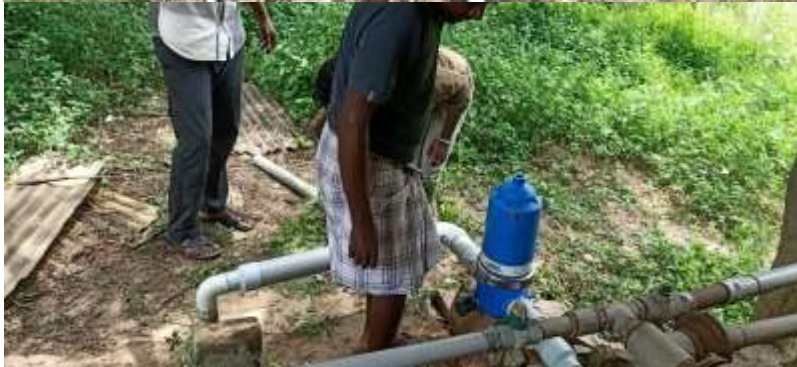
Laying of drip irrigation system in NHM plot
